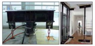
Introduction of "mega piles" for consolidation operation following the foundation collapse of a heavy cemetery building. (Italy 2010)
